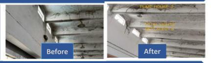
Replacement of 12 Nos 400 W High Bay type HPMV with 135 W highly efficient LED lamp fixture at Compressor House (side of DG Set) in Offsite of Phulpur-II Unit
