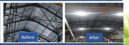
Replacement of 25 Nos 400 W High Bay type HPMV with 135 W high efficient LED lamp fixture at BOP Power Plant of Phulpur-II Unit
