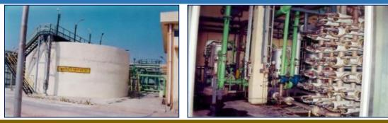
We are using cooling tower blowdown for RO Feed. The recovered RO product is being used in softening plant as make-up water and the reject water is being used in coal yard to supress the coal dust. The Plant Capacity is 3000 M3 /day (Recovery 85 %).
