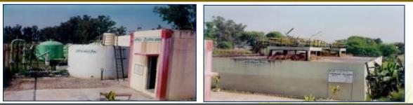
The sewage generated in Plant Township is treated in Sewage Treatment Plant and is being used for irrigation purpose at Farmland at CORDET. The Plant Capacity is 125 M3 / hr.
