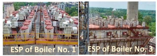
ESP of Coal fired boilers were very old and their performance was deteriorated in due course of time and needed improvement. So, new ESP installed in both Boiler 1 & 3. Installation of ESP of Boiler no. 2 is under progress during the current financial year.
